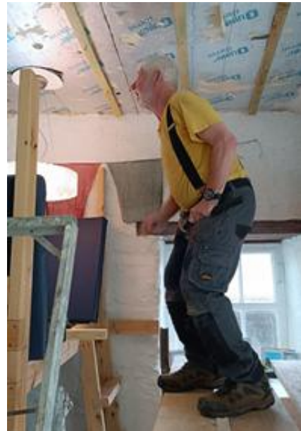
Peter's batten work
