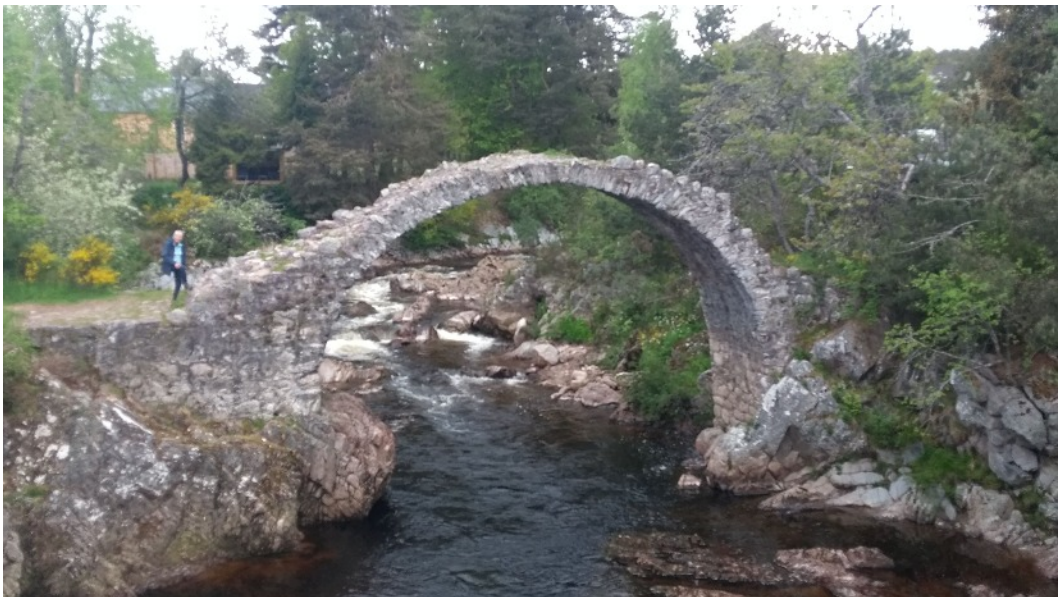
Carrbridge Old Bridge
