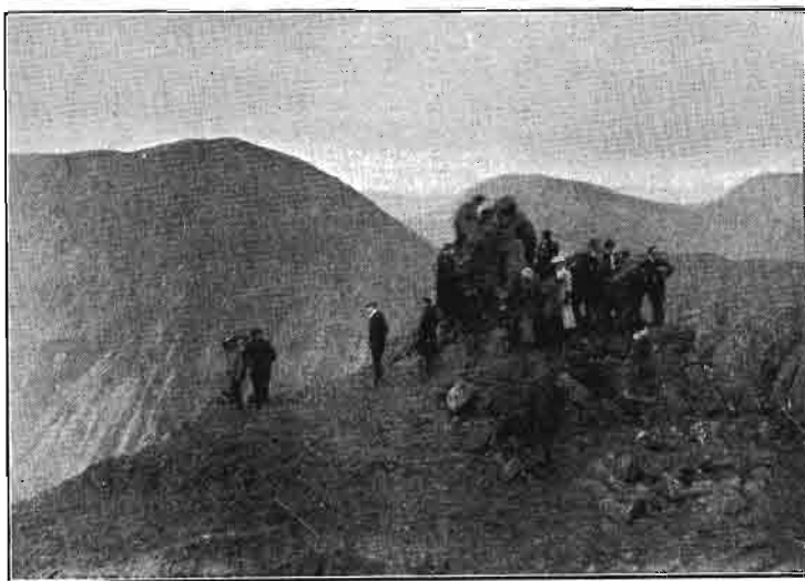
ERECTING THE ROBINSON CAIRN.
