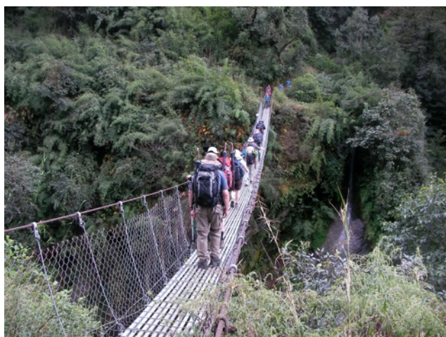
Suspension bridge over the Hinku Khola (MS)
