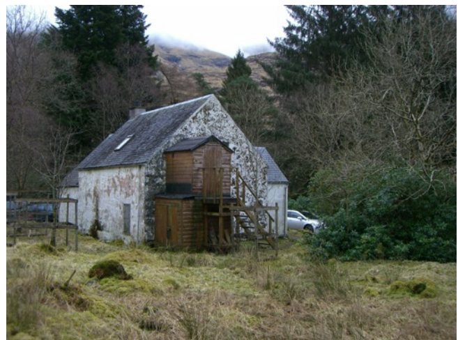
The Grampian Club hut, Inbhirfhaolain photo Adrian Bridge
