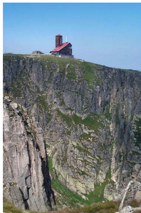
A TV TRANSMITTER STATION HIGH ON THE RIDGE
