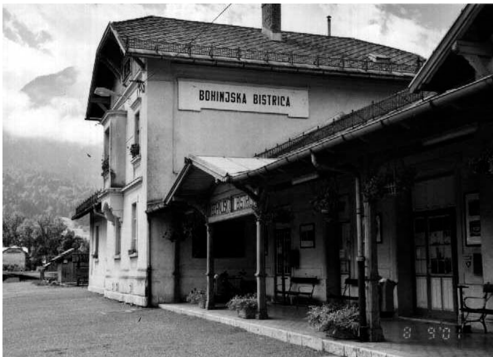
Railway station, Bohinjska Bistrica
