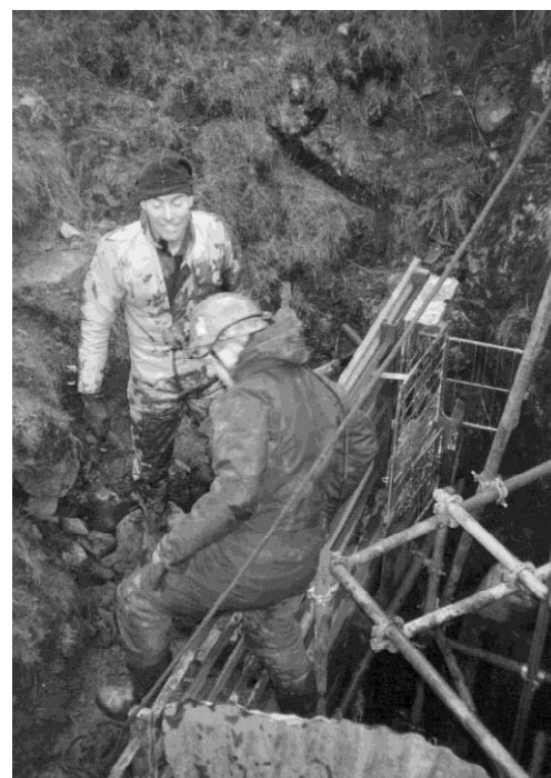
Jed Champion and Robert Crowther during work to improve the security of the passage through the boulders near entrance to the dig on Ingleborough. Photo taken by Michael Smith shortly before the 1999 AGM.
